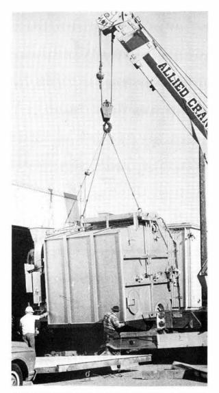
SIXTEEN TONS, and what have you got? A new 16ton boiler for the steam plant, that's what. Installation provides additional capability, serves as backup to existing boilers.
